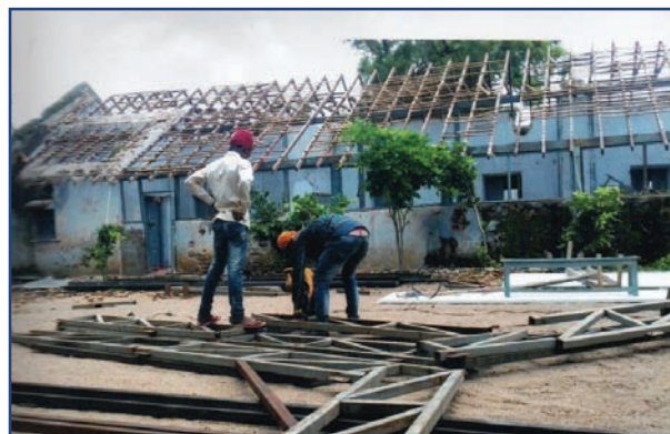
Kasturi Foundation, Hyderabad Repairing the School Building
