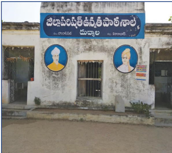
The condition of the school till 2017
