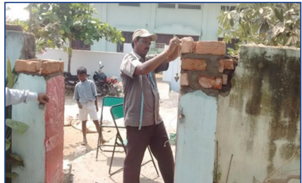
SMC chairman G.Rambabu Constructing School board pillar voluntarily
